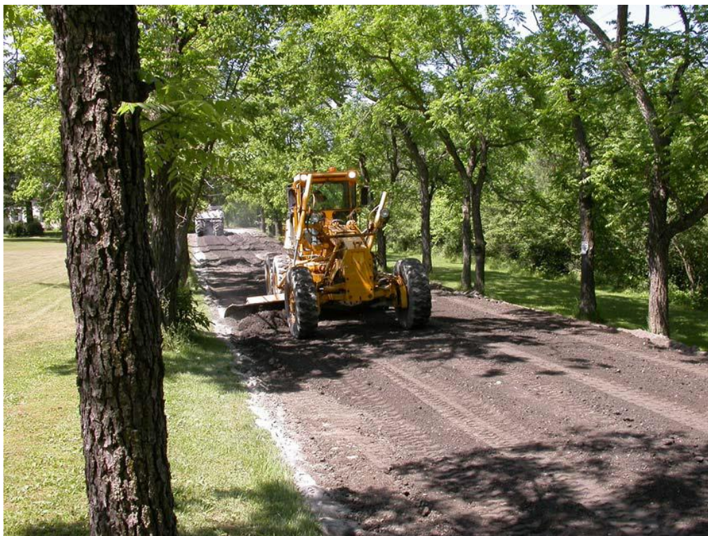
Figure 2:4: Initial shaping with motor grader (Morian et al. 2012)
