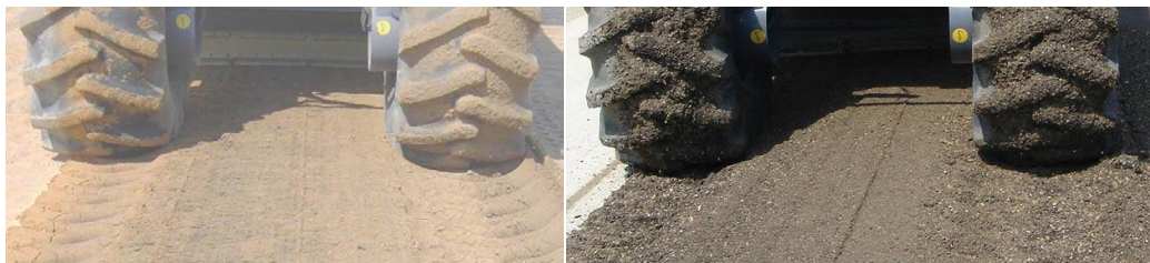
Figure 2:7: Observation behind the recycler: (left) emulsion, (right) foam (Asphalt Academy 2009)
